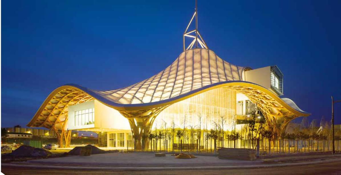
Shigeru's Pompidou of the South's roof structure is composed of timber that intersect to form hexagonal wooden units resembling the cane-work pattern of a Chinese hat (see design detail opposite).
